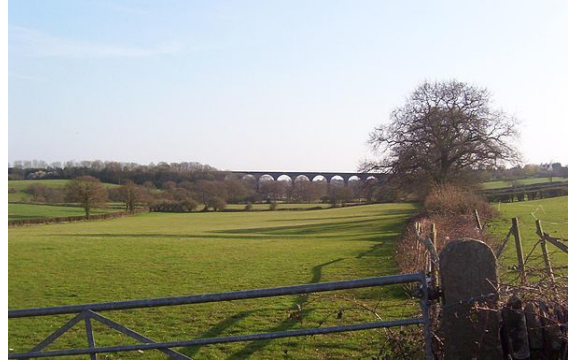
Looking towards the Huckford Viaduct and Frome Valley from Cloisters
